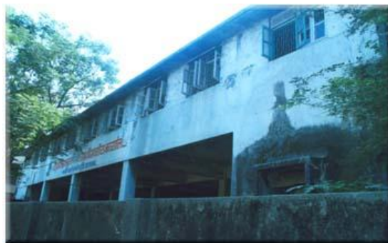
Inspector Office, Raigad Region, Panvel (022)22923528, Fax:27451205
